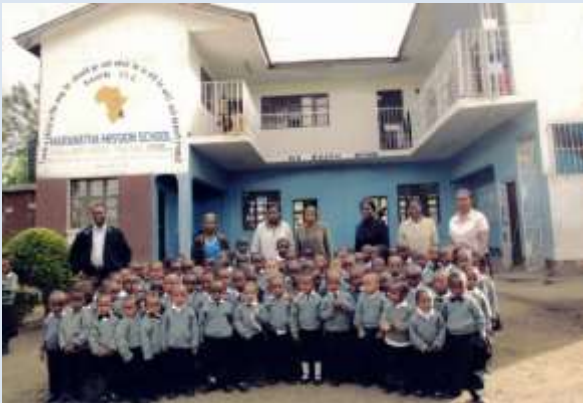
Original building ,after adding second story
