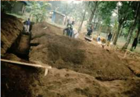
Clearing the land and starting the foundation
