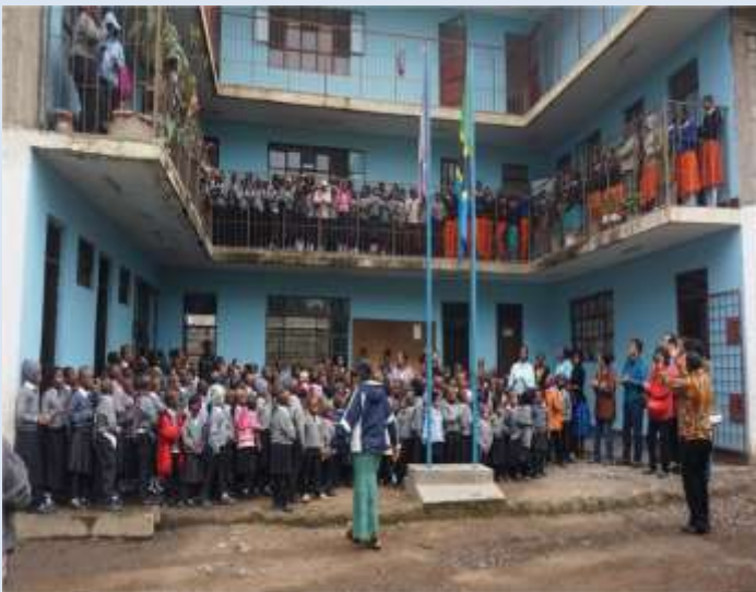
Current building used for Elementary School
